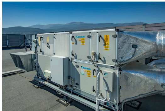
Air handling units guarantee fresh air supply at the pool, the gym, and the spa.
