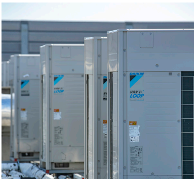
Thanks to 300 VRV heat recovery systems (outdoor units' capacity: 3500 HP), no gas heating system is needed.
