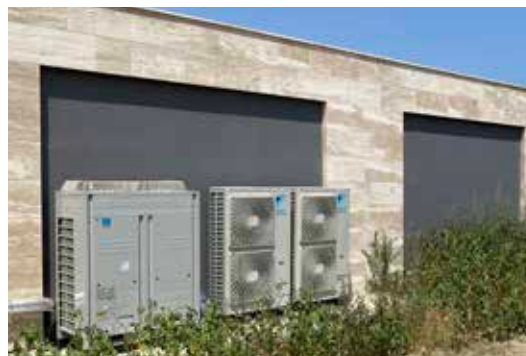
VRV and ZEAS outdoor units are located away from the main hotel to minimise disturbance.
